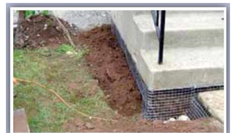
L-Shaped screen application around foundation.**
