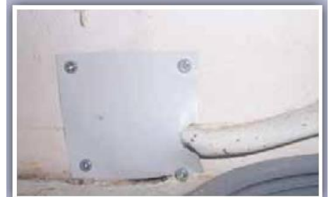
Power supply hole sealed with metal flashing.*
