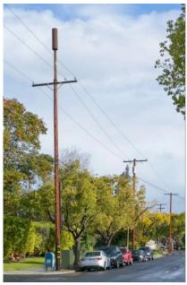
(B) Below is an example of an acceptable radio and antenna strand-mounted on aerial fiber optic cable:
