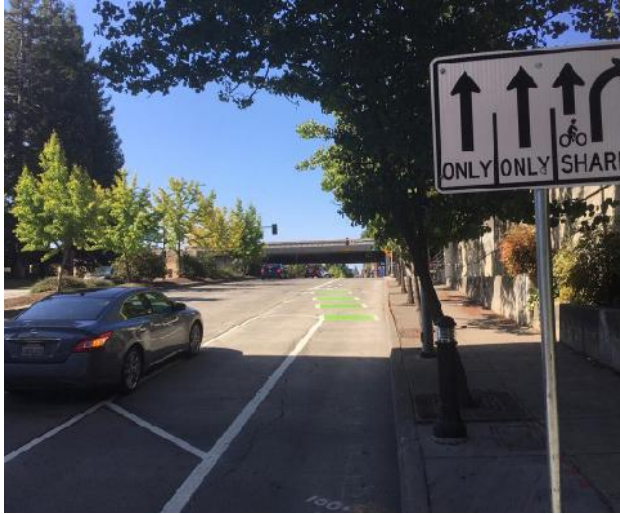
Buffered bike lanes transition into conflict markings.
