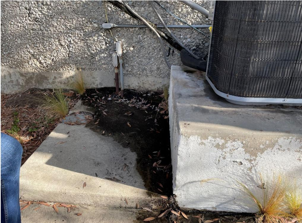
Photo 9: Water leak and possible mold growth near first floor air conditioning system.
