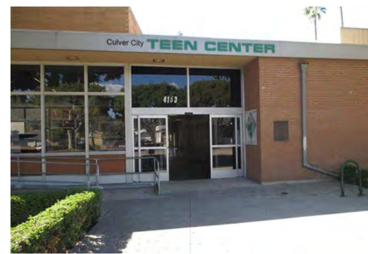
SUBSTANDARD TEEN CENTER BUILDING
