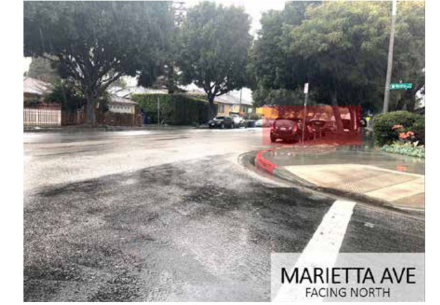
Existing condition of parking and parkway landscaping on east side of Elenda St between Marietta Ave and Arizona Ave interferes with the clear sight triangles for vehicles turning right or left onto Elenda St.
