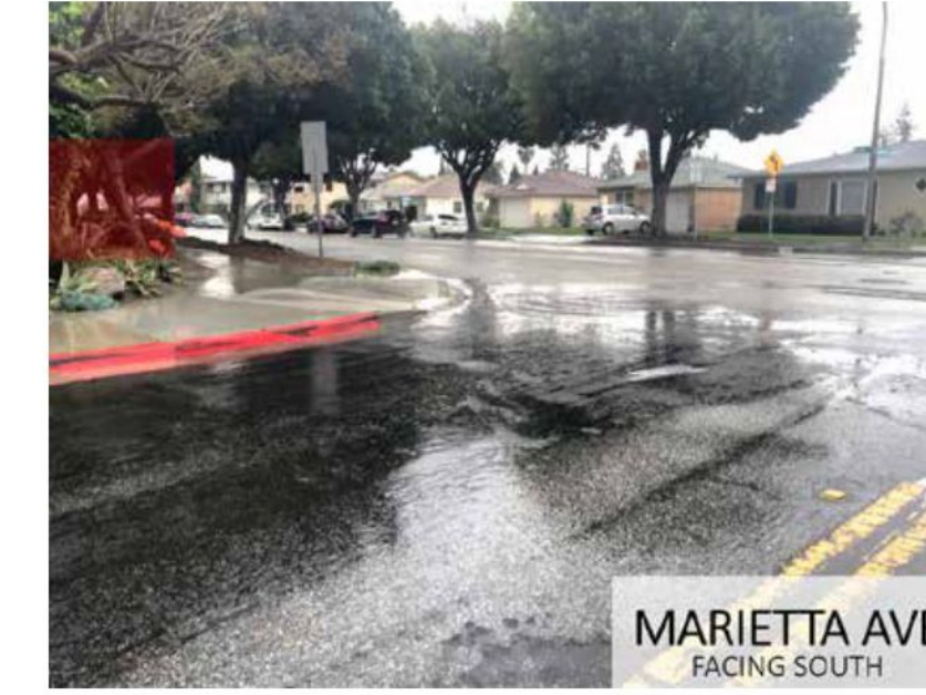
Existing condition of parkway landscaping and curvature of Elenda St between Marietta Ave and Culver Blvd interferes with the clear sight triangles for vehicles turning right or left onto Elenda St.
